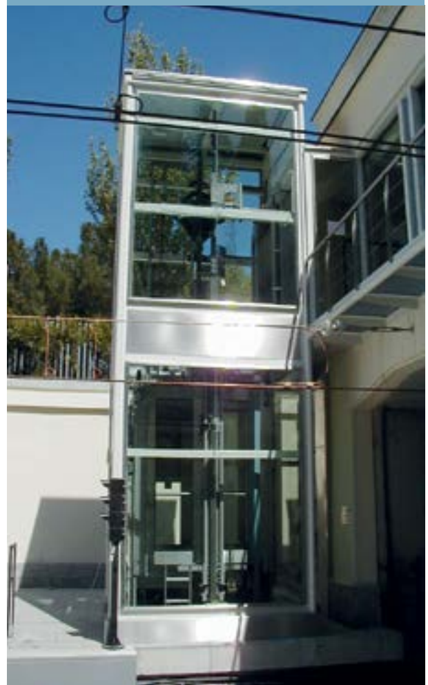
Figure 3. Self-standing steel shaft
